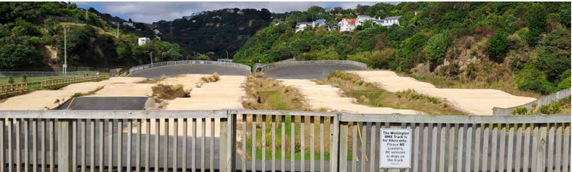
Image above: Completed BMX track upgrade.
